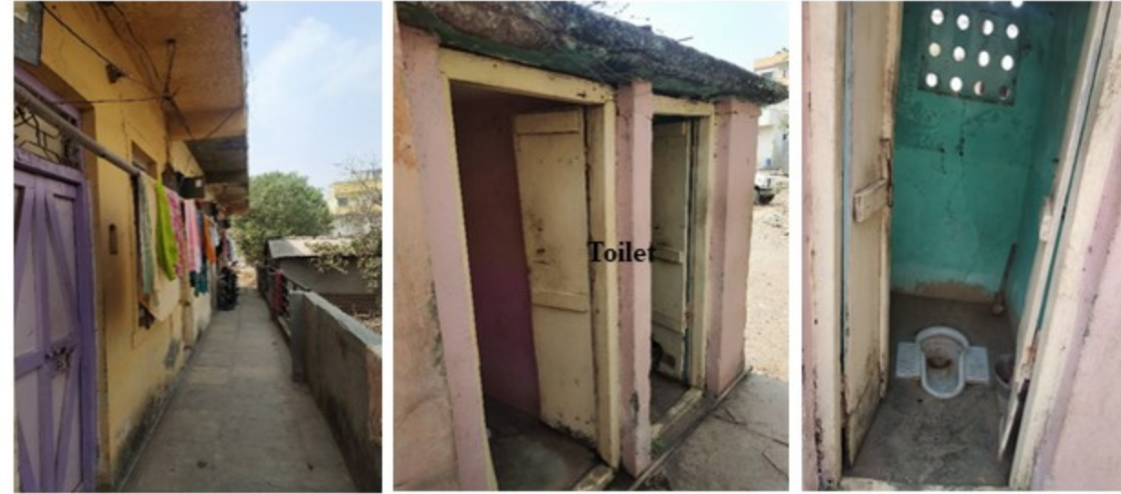
Six Superstructures with two group toilet connected to septic tank
