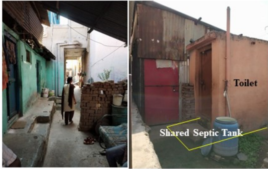
Three Superstructures with one group toilet + septic tank
