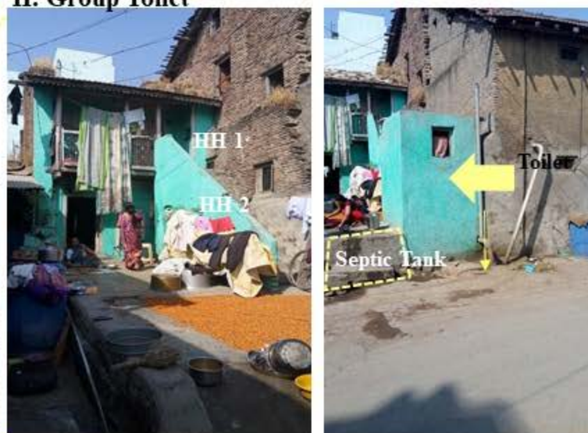
Two Superstructures with one group toilet + septic tank
